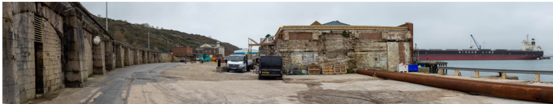
Two views along the lower level of the breakwater showing the coal storage casements
