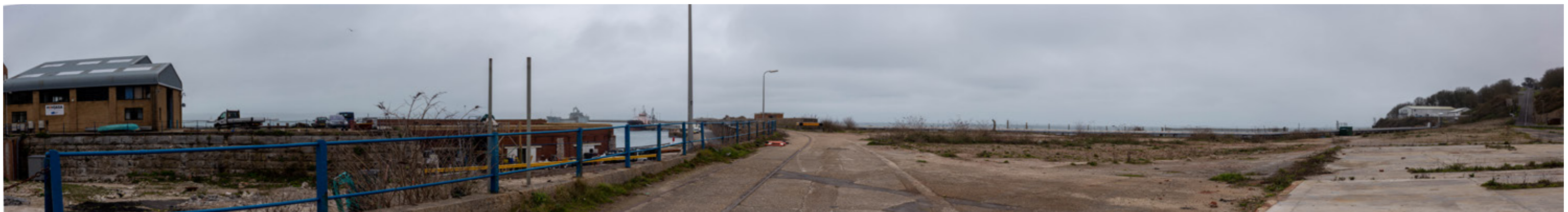
View along the upper level of the breakwater
